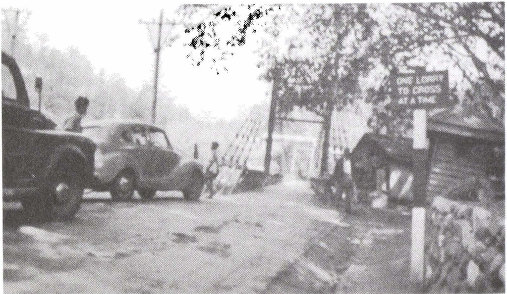
The Rongpo bridge into Sikkim (1955)
